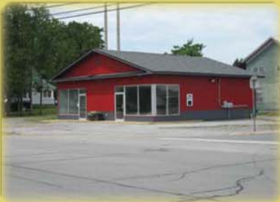
Former Alaskan Oil/Marino's
