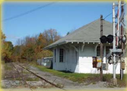
Train Station / Agway Property
